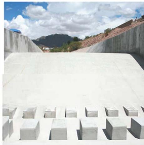
The Bear Ridge Channel was changed to increase its capacity, and energy dissipaters were added to reduce the speed of stormwater gushing from the Franklin Mountains.
